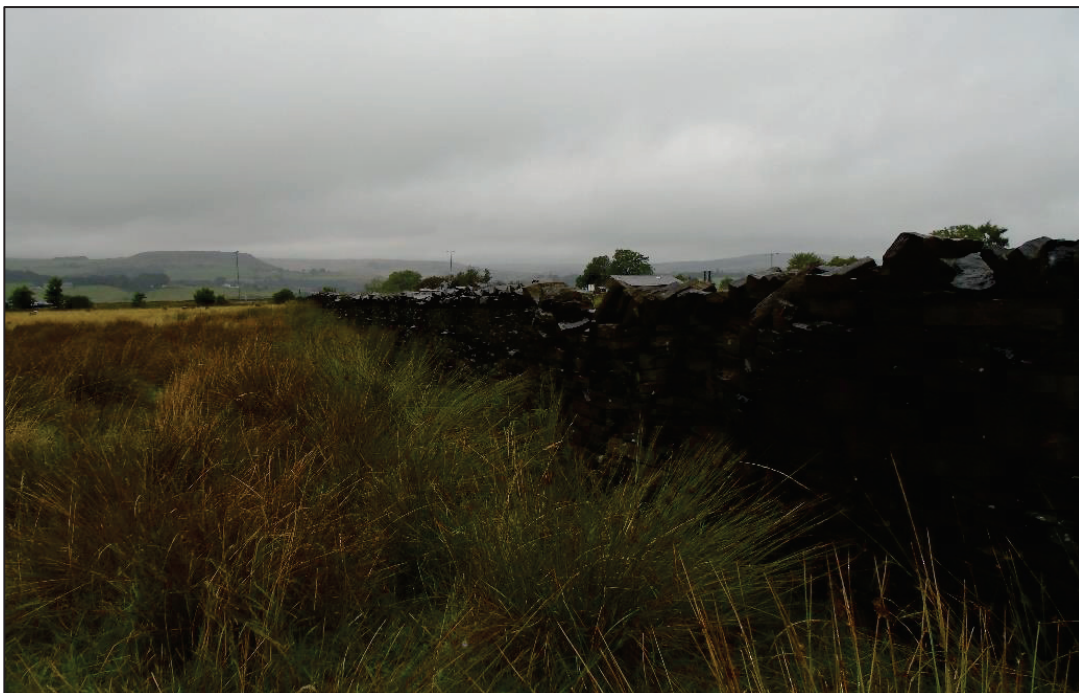
Figure 10: Dry stone wall along the northern boundary of the proposed site.
