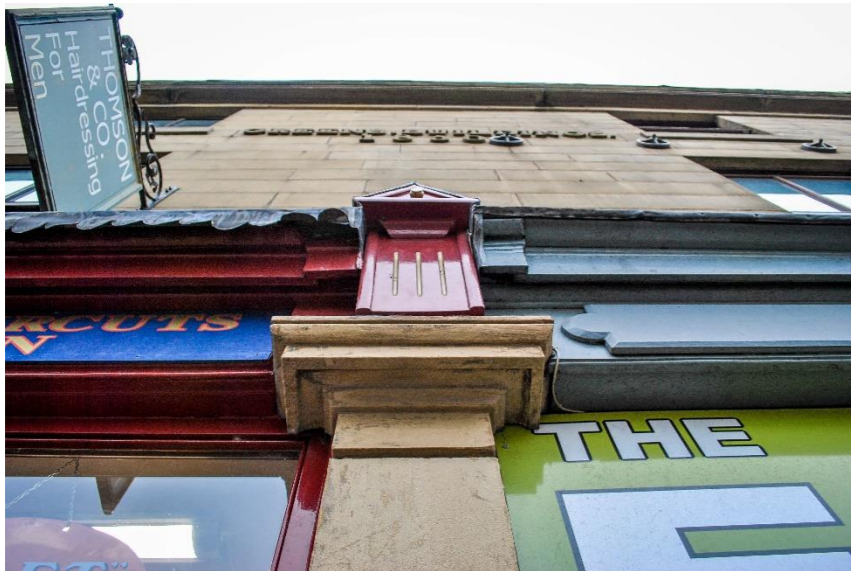
Figure 97 Thomson Barber Shop, 63 Deardengate - detail
