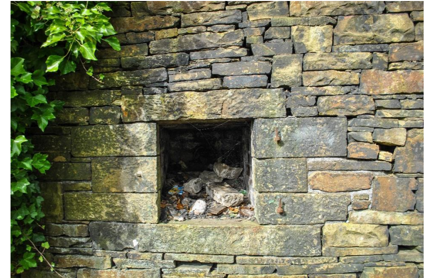
Figure 32 Feature of historic wall on Bell Street
