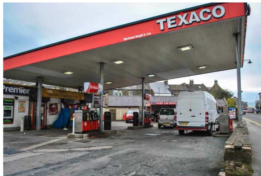
Figure 90 Petrol Station Forecourt
