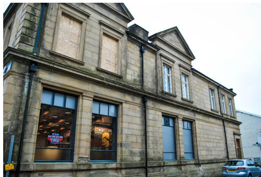
Figure 86 67 Deardengate from Ratcliffe Street
