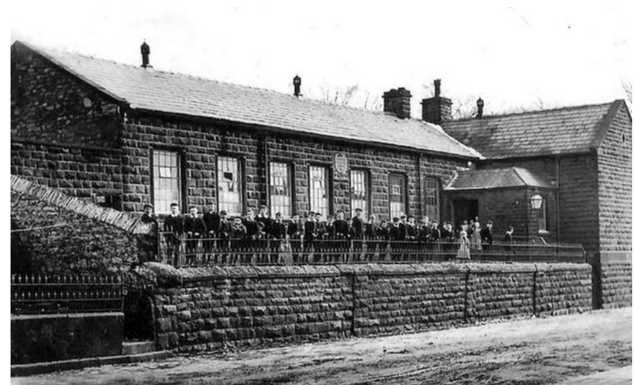
Figure 4.19: An undated photograph of the former National School and Sunday School, Burnley Road
