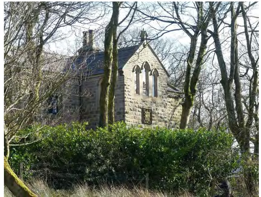
Figure 4.11: The entrance wing to the western elevation
