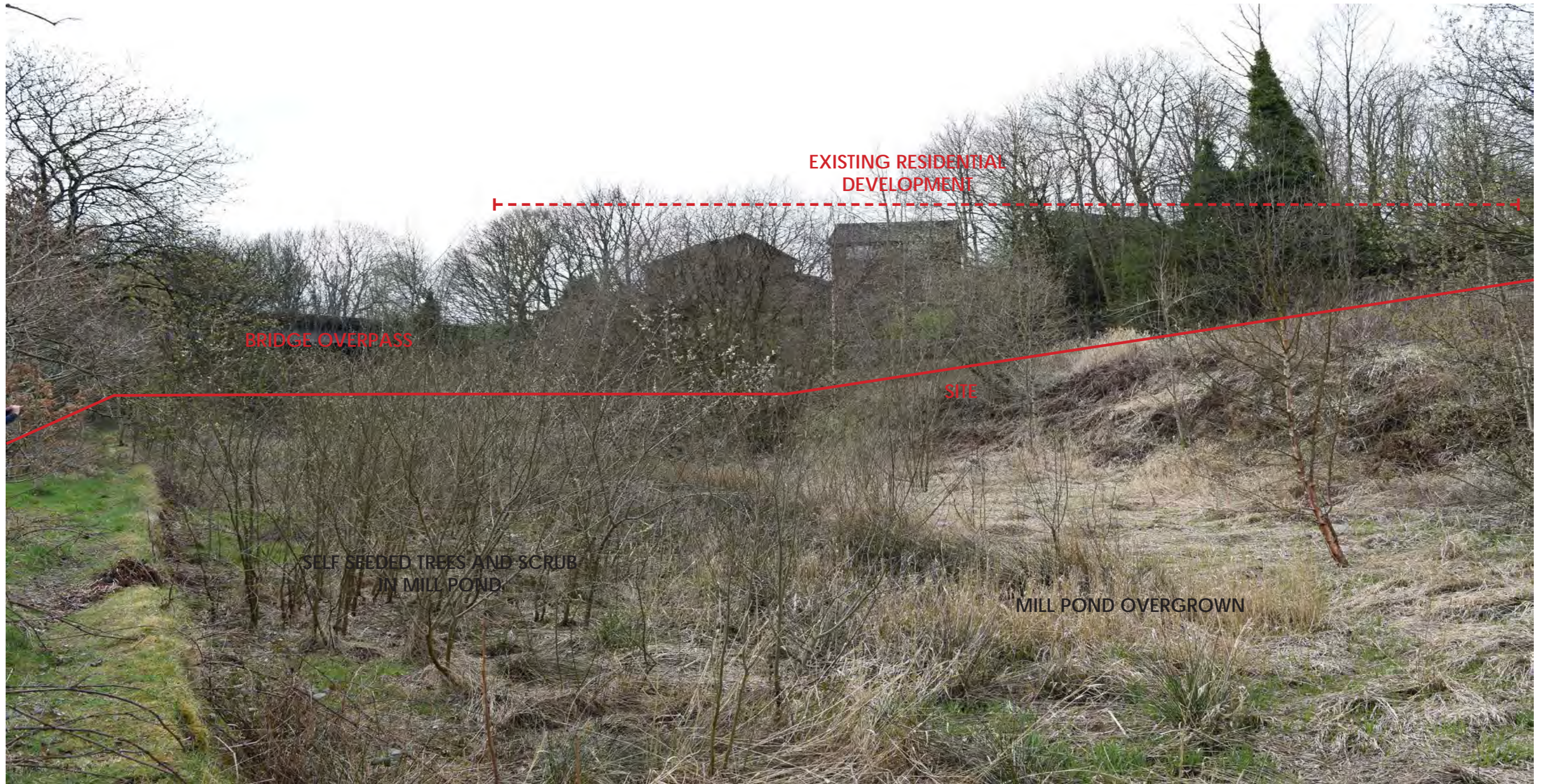
VIEW LOOKING SOUTH WEST FROM TOP OF MILL POND WALL
