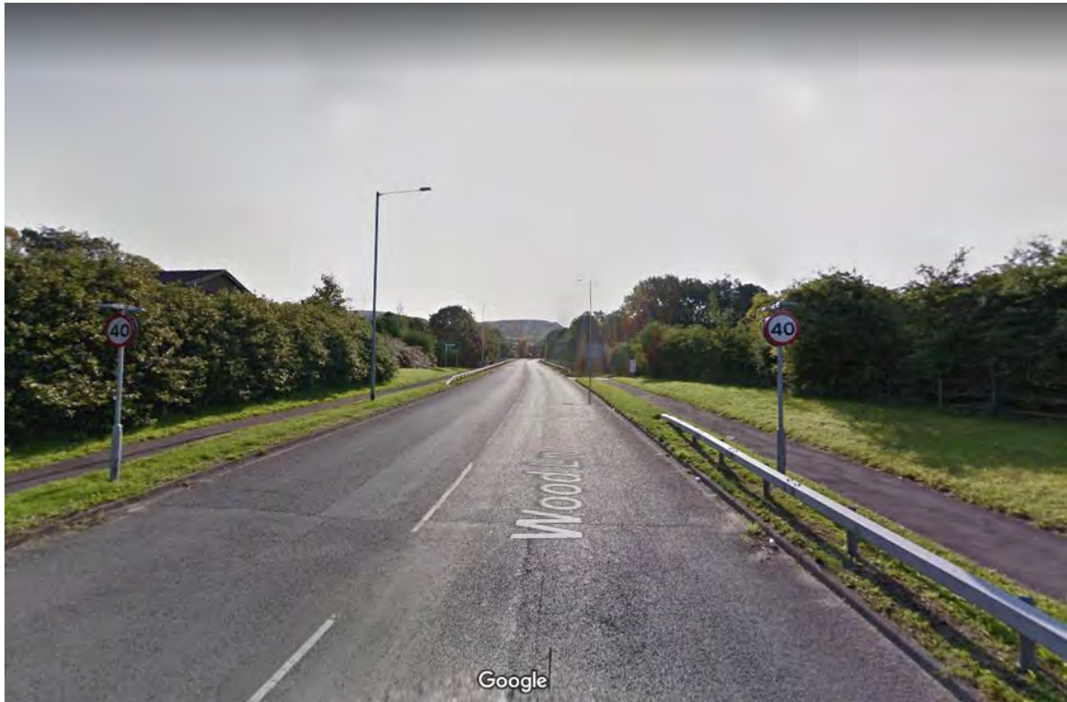
Figure 4: Wood Lane (Looking East)
