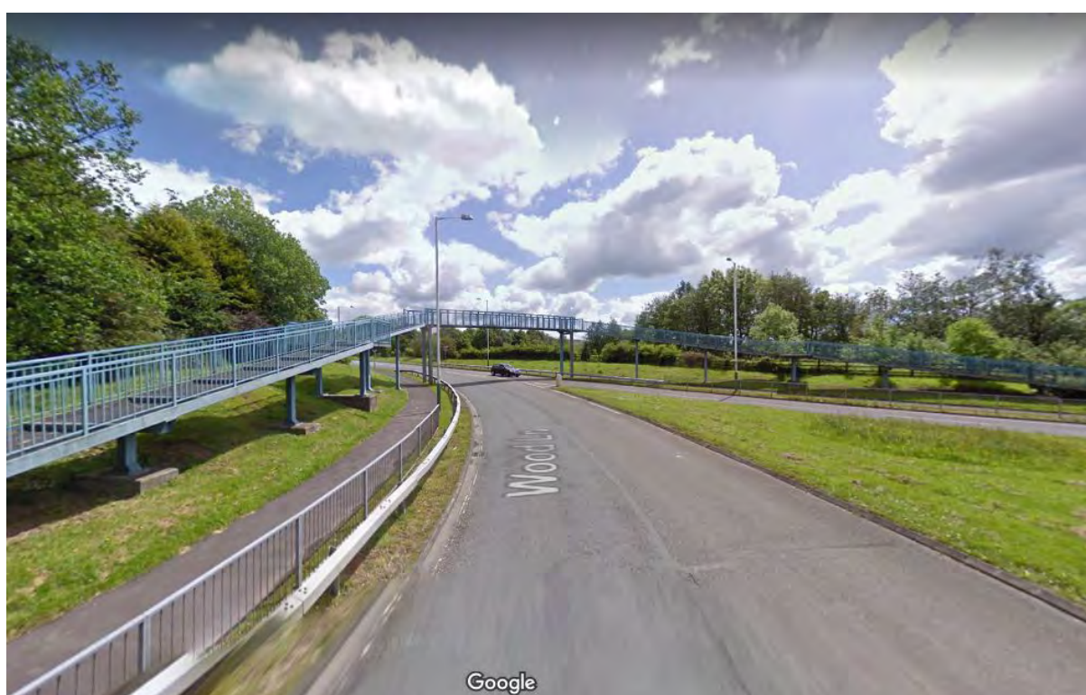
Figure 2: A56 Wood Lane Pedestrian Overbridge
