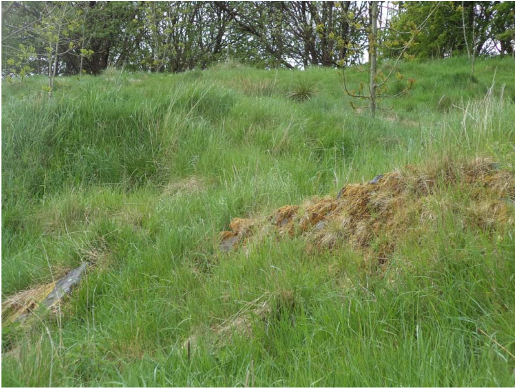
Photograph 19 Demolition debris in the old sewage settlement tanks in the northern site area
