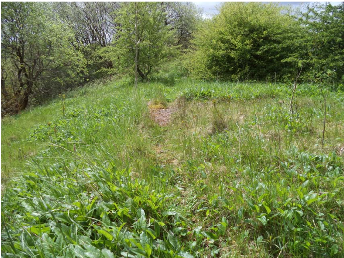
Photograph 16 Southern area of site with demolished structure close to the centre of the photograph
