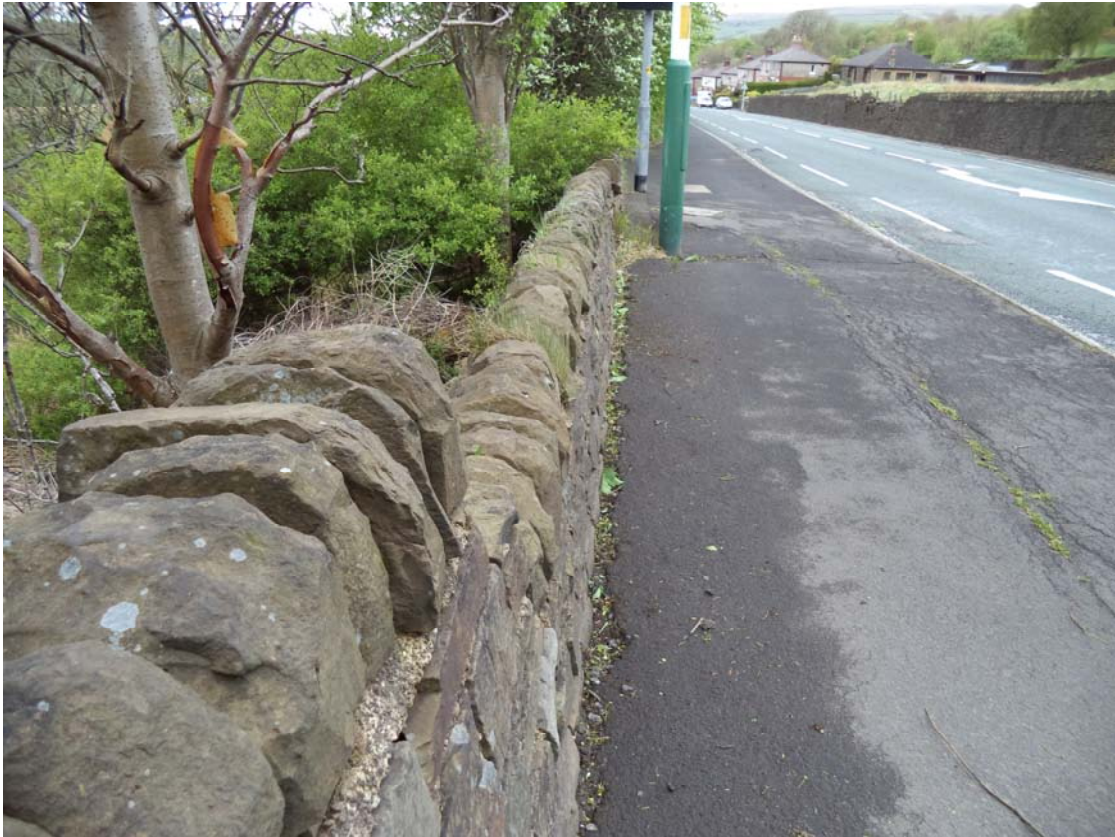
Photograph 21 Steep slope in southern area of site looking southwards to property on Hillside Drive
