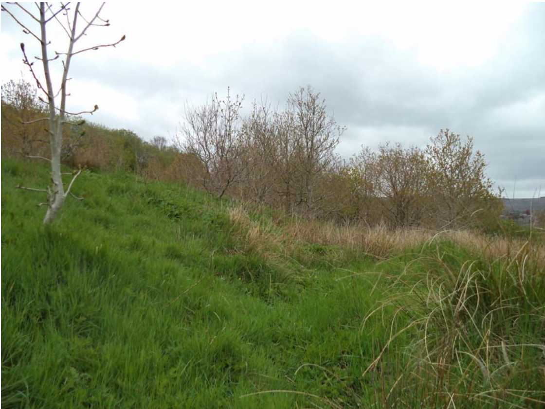
Photograph 12 Base of western slip scar in central area of site looking northwards
