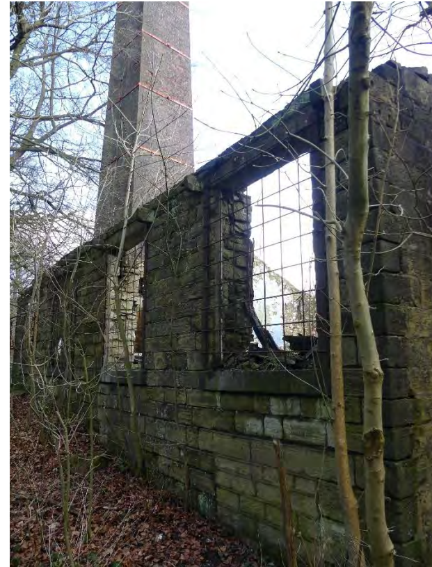
Figure 3.11: The western elevation of the single storey range to the lane
