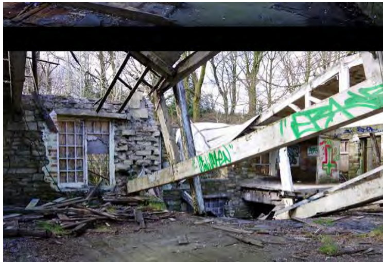
Figure 3.13: Collapsed trusses in the early C19th range ( luigidawn.blogspot.com )
