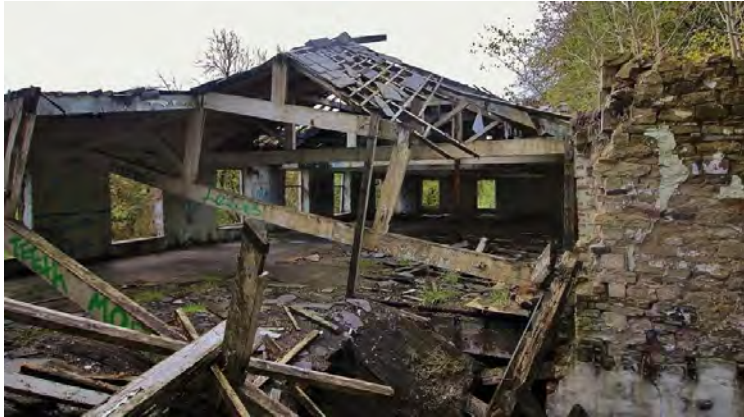
Figure 3.13: Collapsed trusses in the early C19th range ( luigidawn.blogspot.com )
