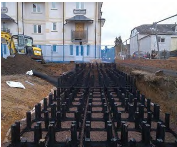
Figure 3 Buckland House Car Park construction phase (1)
