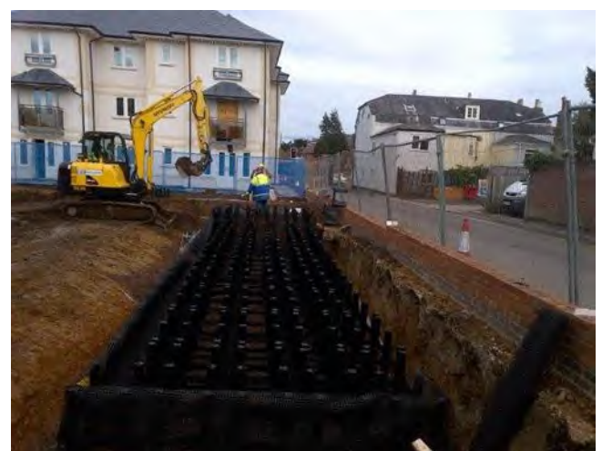
Figure 4 Buckland House Car Park construction phase (2)
