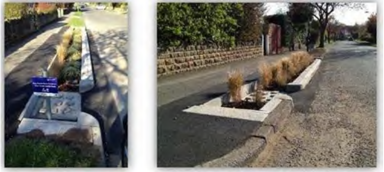
Figure 6 Completed rain gardens (2)
