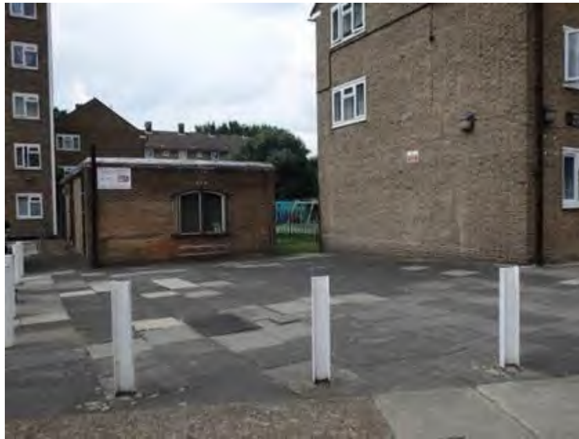
Figure 1 Prior to SuDS construction
