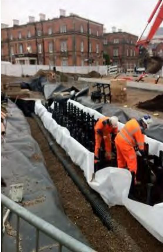
Figure 2 Construction of tree pit
