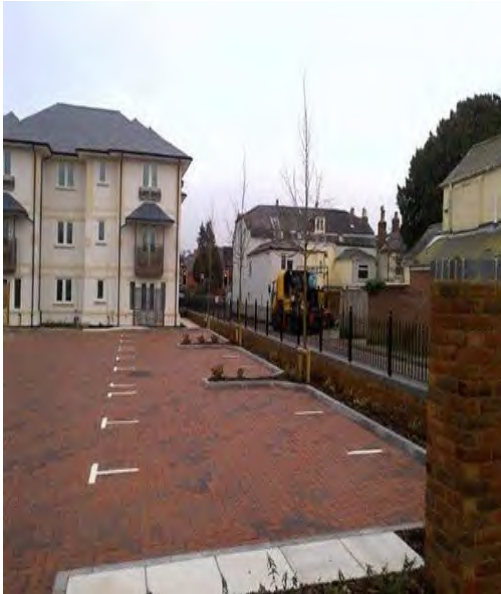
Figure 1 Buckland House Car Park (1)
