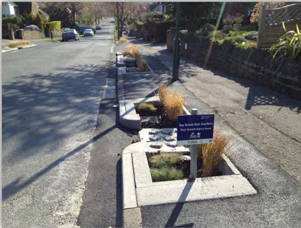
Figure 5 Completed rain gardens (1)
