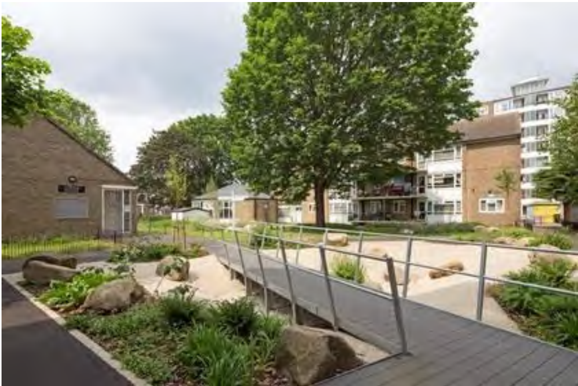
Figure 6 Stony detention basin
