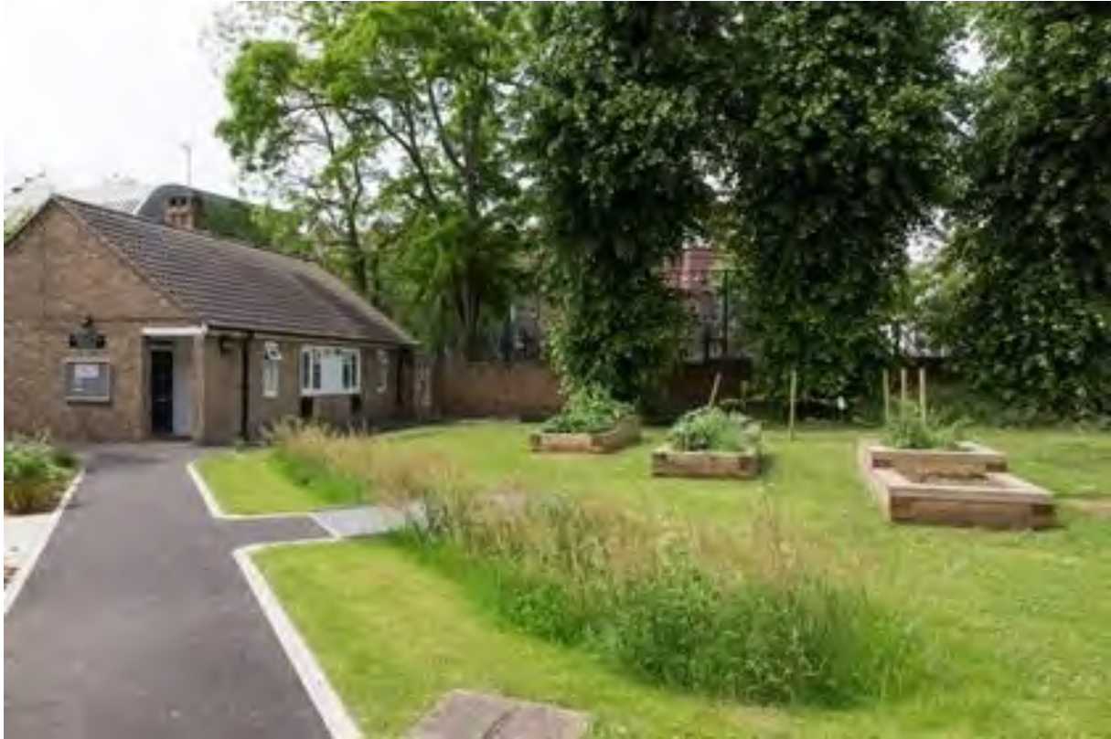
Figure 7 Swale and food growing
