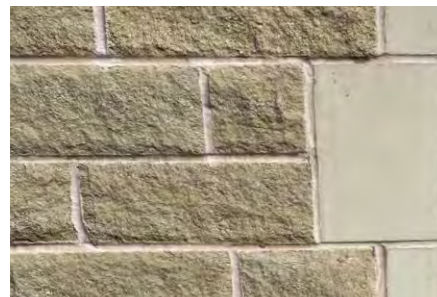
Fig 3.3 Stone effect/reconstituted stone brickwork
