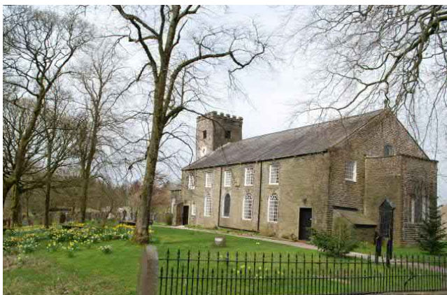
Edenfield Parish Church, located in Village Core A
