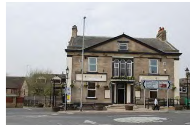
Rostron Arms, located in Village Core B
