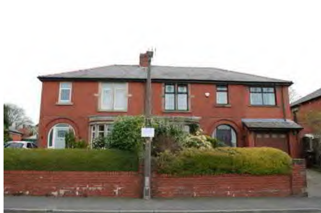
Post-war red brick semi-detached domestic development
