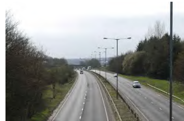
View looking south down the A56/ M66
