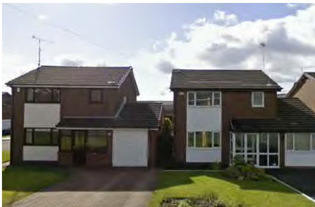
Detached development within domestic character area
