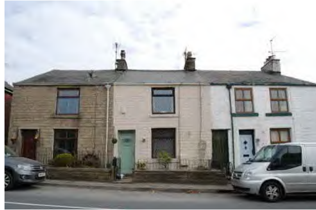
Traditional Terraces with low boundary wall and minimum setback
