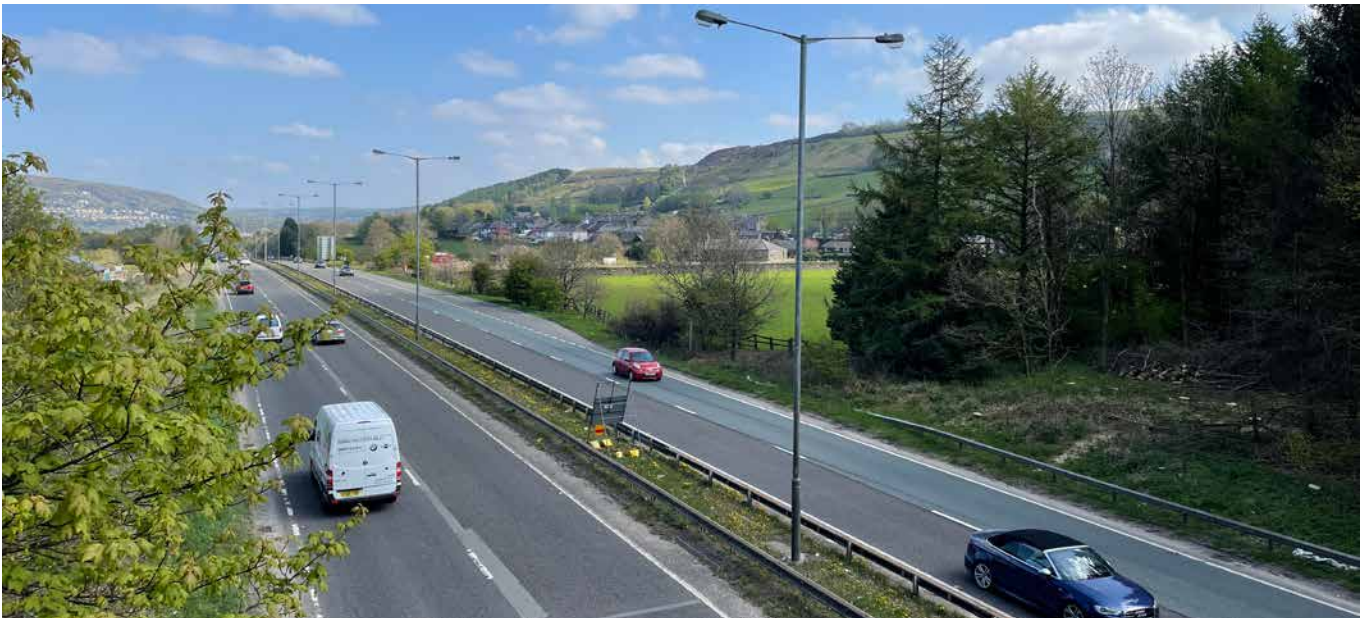
A56 - dual carriageway
