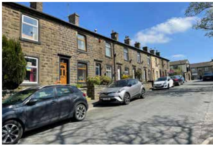
Strong build line along Exchange Street
