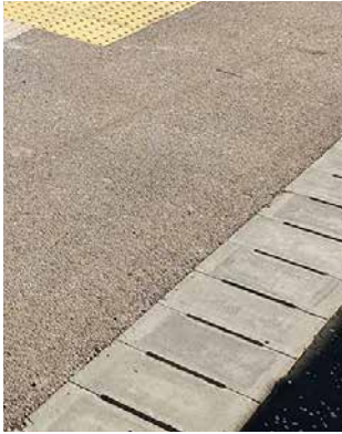
Range of indicative landscaping and surfacing details which may be appropriate for use (details to be agreed with LPA)
