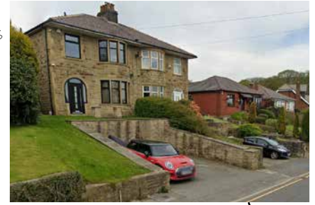
Stone faced retaining walls
