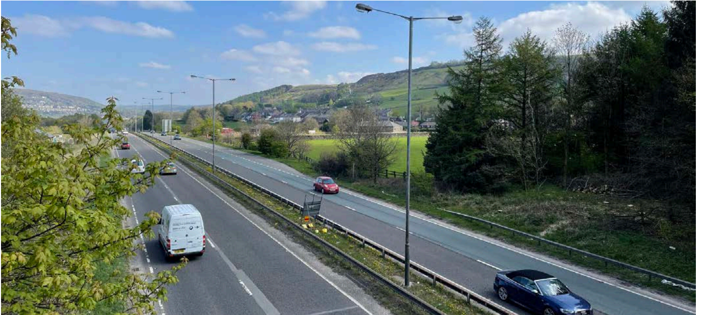
A56 - dual carriageway
