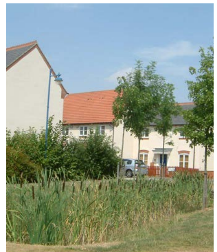
Example SUDS swale with reed bed
