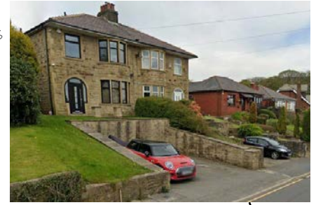
Stone faced retaining walls
