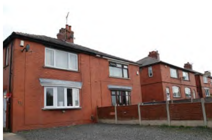
Red brick domestic style with low levels of detailing
