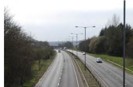
View looking south down the A56/ M6
