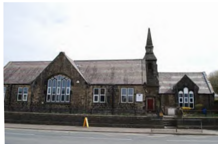
Edenfield Church of England Primary School, located in Village Core A
