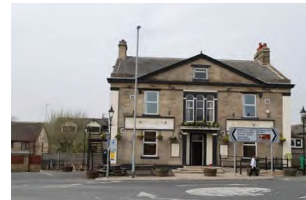
Rostron Arms, located in Village Core B
