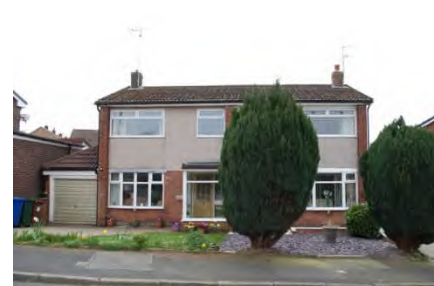
Different application of external material on first and ground floor facade
