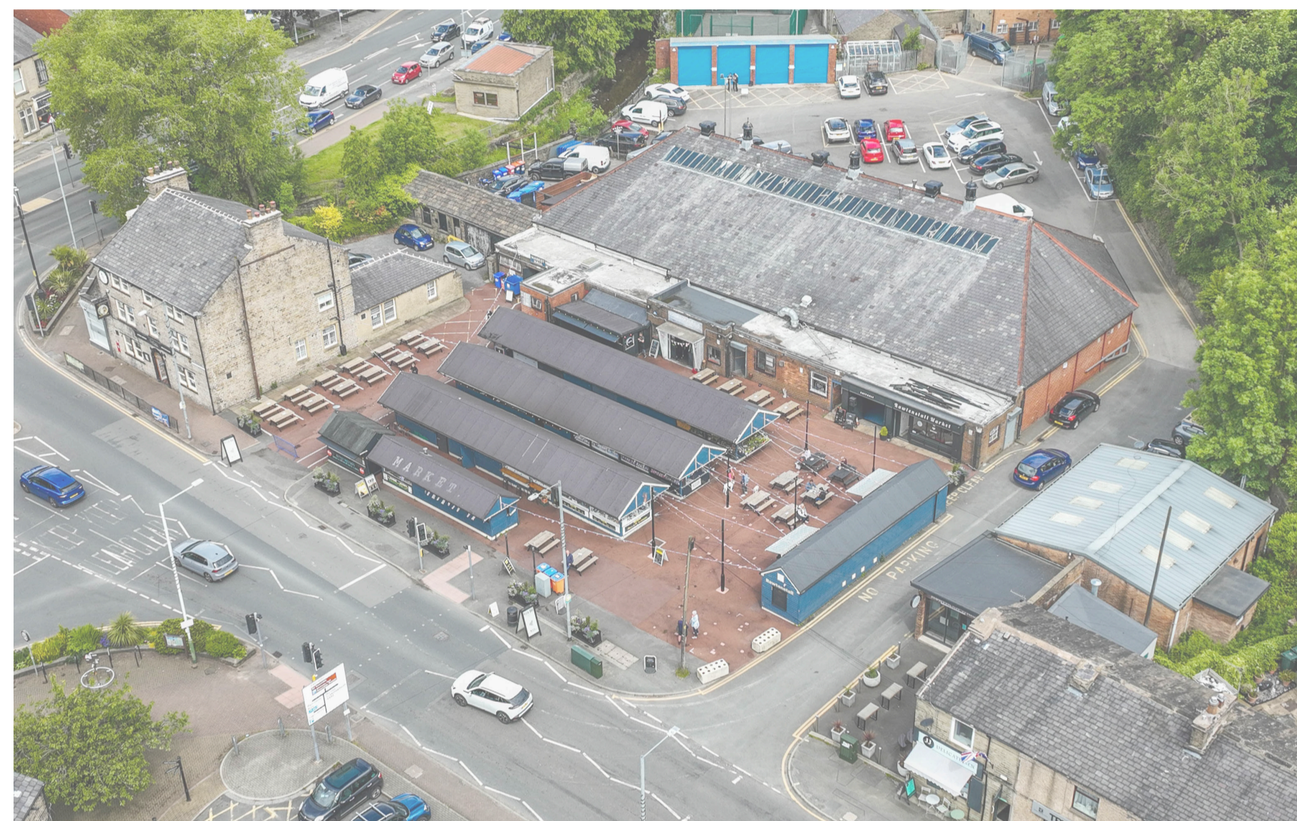
Aerial View of Existing Site
