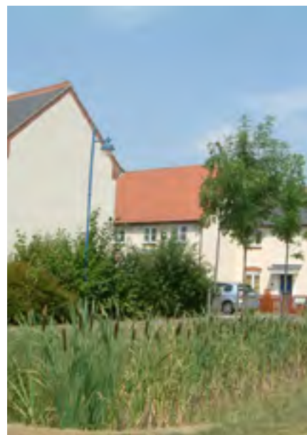
Example SUDS swale with reed bed
