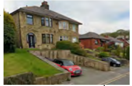
Stone faced retaining walls
