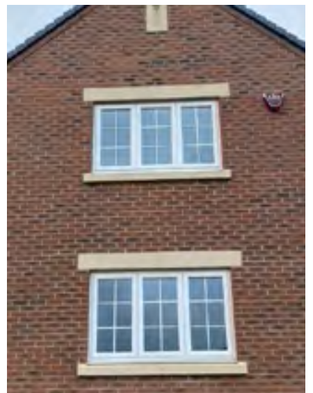
Stone cill and header detail
