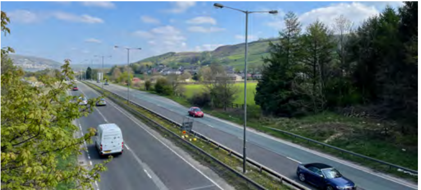
A56 - dual carriageway
