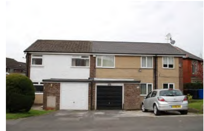
Painted brick finish post-war domestic development
