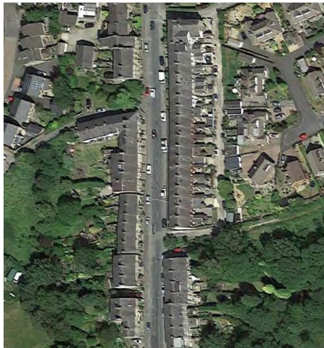
High density structure of Traditional Terraces AECOM
