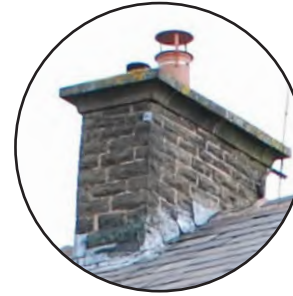
Chimneys help to add rhythm to the streetscape and are a key characteristic of the local area
