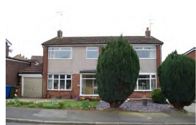
Different application of external material on first and ground floor facade
