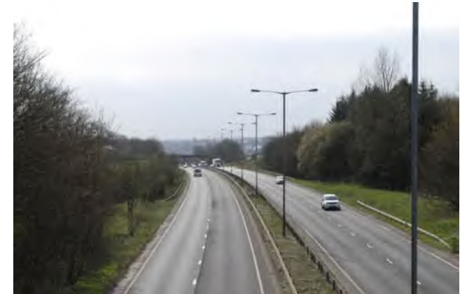
View looking south down the A56/ M66
