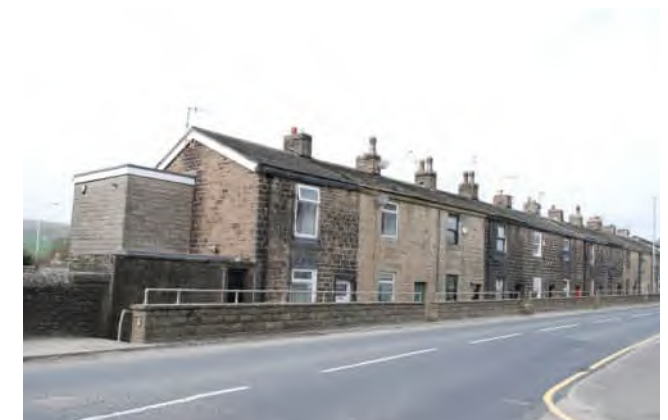
Continuous row of traditional terraces along street
