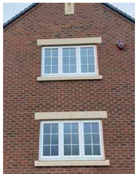
Stone cill and header detail
