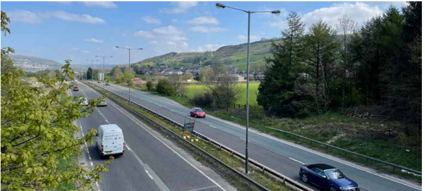
A56 - dual carriageway
