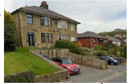
Stone faced retaining walls
