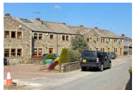
Hard standing areas of frontage parking
