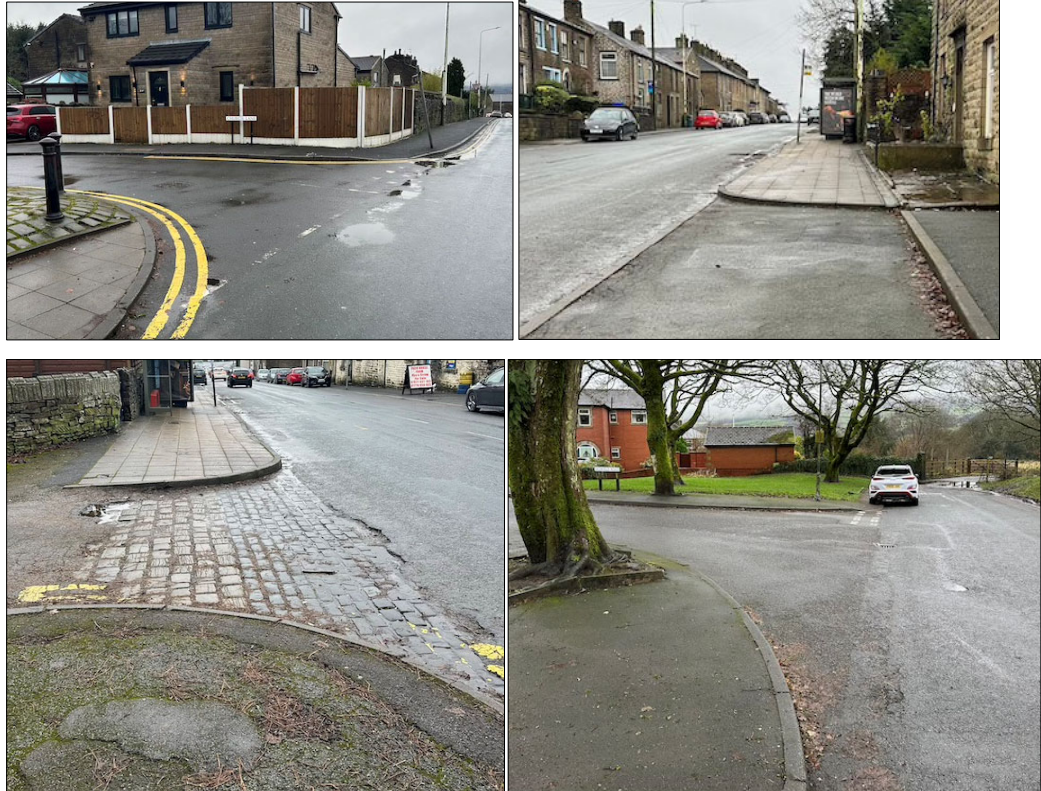
Photographs 3-6 – Examples of deficiencies in uncontrolled pedestrian crossing provision.
