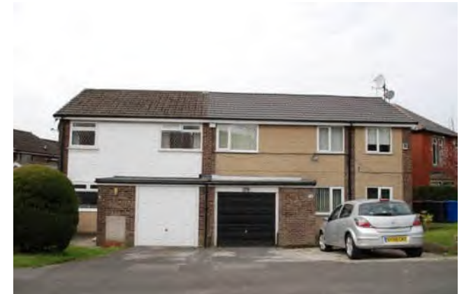
Painted brick finish post-war domestic development
