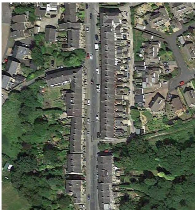
High density structure of Traditional Terraces AECOM
