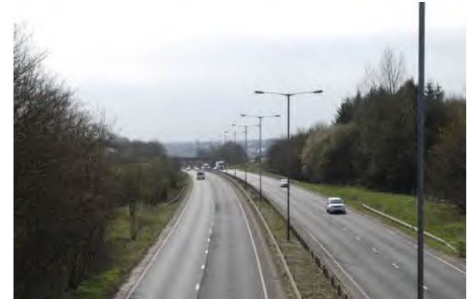
View looking south down the A56/ M66
