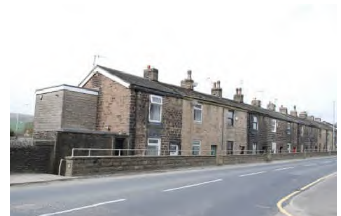
Continuous row of traditional terraces along street
