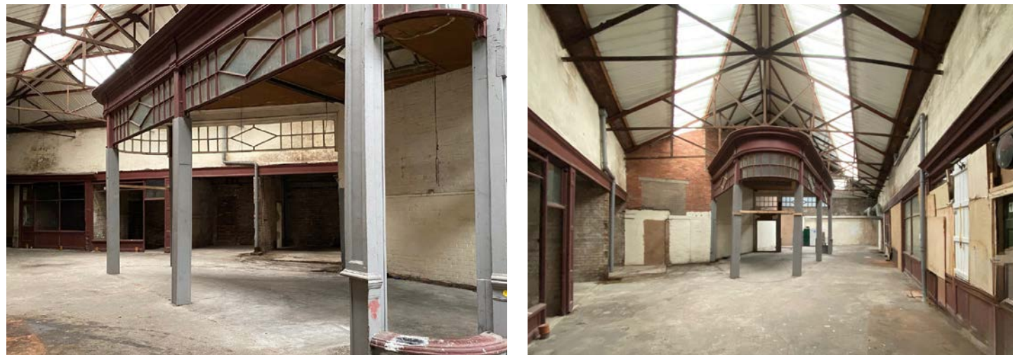
EXISTING INTERNAL ARCADE:
