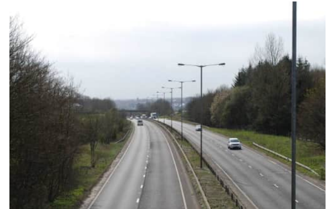
View looking south down the A56/ M66
