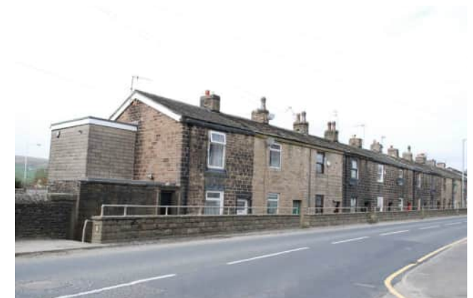
Continuous row of traditional terraces along street
