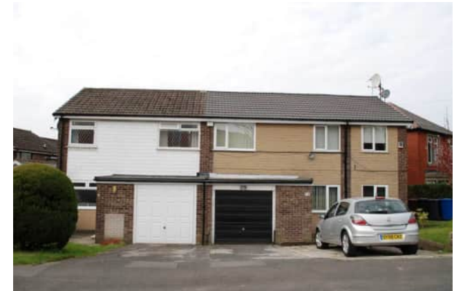
Painted brick finish post-war domestic development
