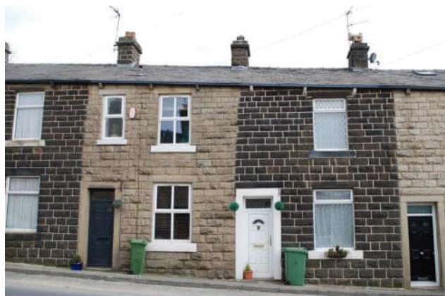
Different coloured Pennine stone facade adding to the local character
